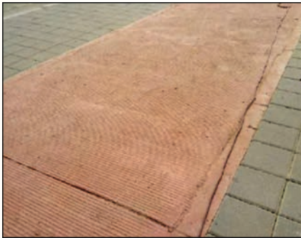
Fig 8: Concrete Broomed Surface/ Concrete Tiles
