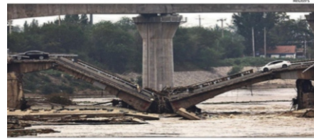
A highway bridge in Heilongjiang province collapsed on Thursday due to flash floods triggered by heavy rains as parts of China experience the worst floods in decades. Two cars fell into the Mayi river, but no casualties were reported. A rescue operation was ongoing, and a section of the highway was closed, according to state media. On Wednesday, authorities said Beijing recorded its heaviest rainfall in at least 140 years over the past few days as remnants of typhoon Doksuri deluged the region.
