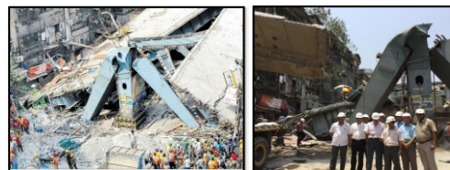
Vivekananda Flyover under construction by KMDA, Govt. of West Bengal. Suddenly collapsed on 31.03.2016
