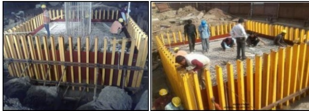
Protection of worksite... (Pile Cap work)
